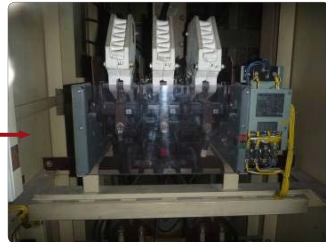
Installing the insulation to the bus bars
