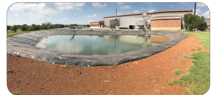
First flush containment pond
