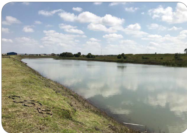
First flush containment pond
